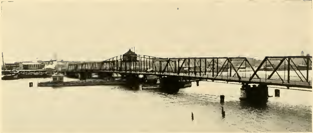
THIRD STREET BRIDGE
